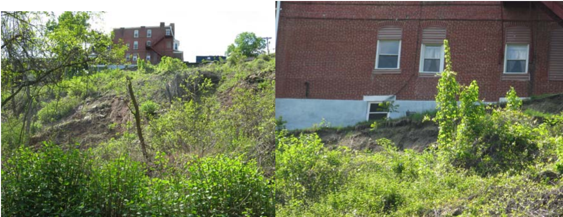
Oakland Square – building too close to a steep slope can be dangerous if that slope fails, as it has in this case
